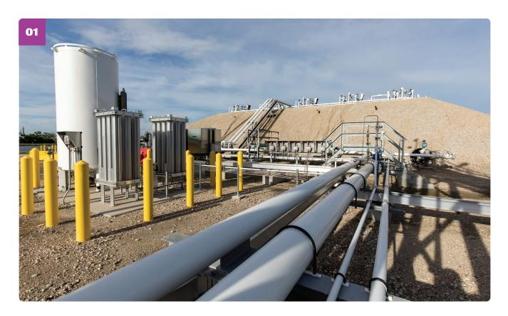
AS PART of the Vopak Moda Houston project, EPC contractor Transtech Energy, which has over 30 years of experience in the design and construction of liquefied gas terminals and transloading facilities, was tasked with fabrication of the facility's five pressurised 120,000 gallon bullet tanks. These tanks have a total storage capacity of 14,285 barrels for products such as propane or butane or other liquefied hydrocarbon gasses.
