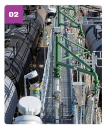
As part of their scope Transtech Energy also engineered and built the rail terminal. 'When designing this, we had to ensure the rail access platform system was expandable to handle additional rail cars for potential growth of the facility,' says Wenik. 'The initial design allows for the unloading of multiple railcars
